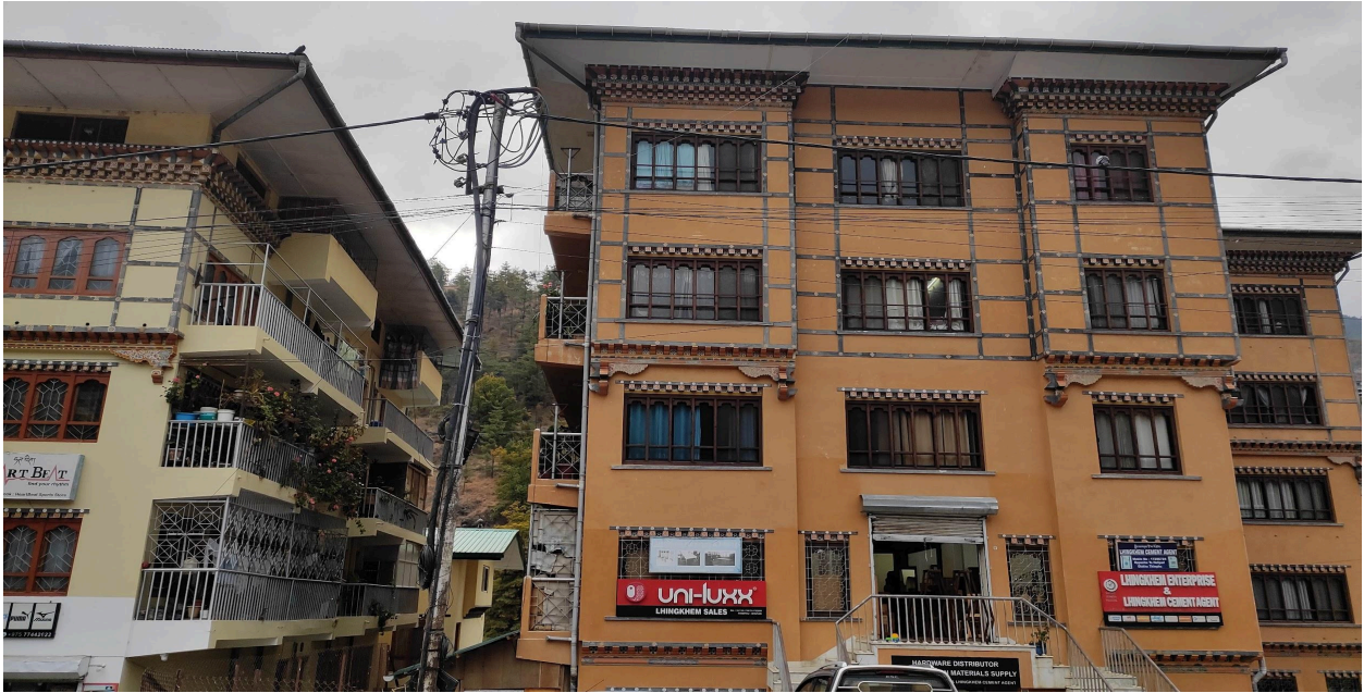
Figure 8: Improper cable layout at Changjalu, Before and After
