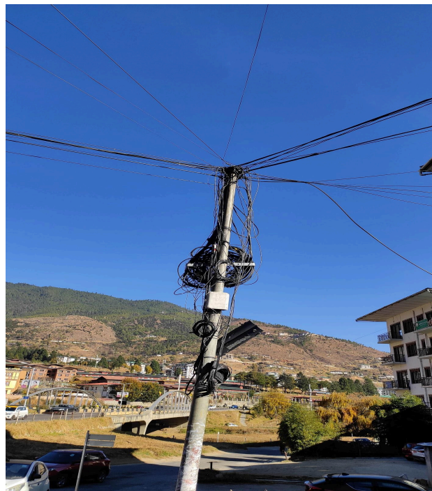
Figure 10: Improper crisscrossing of cables at Changbangdu, Before and After
