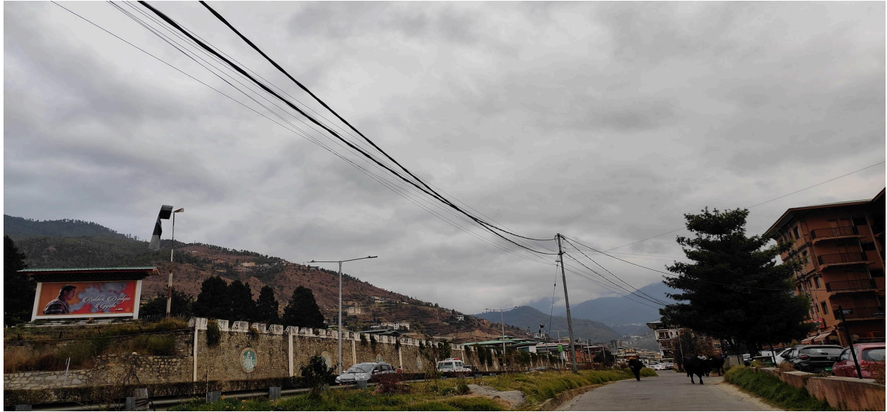
Figure 9: Improper cable layout near Helipad, Before and After
