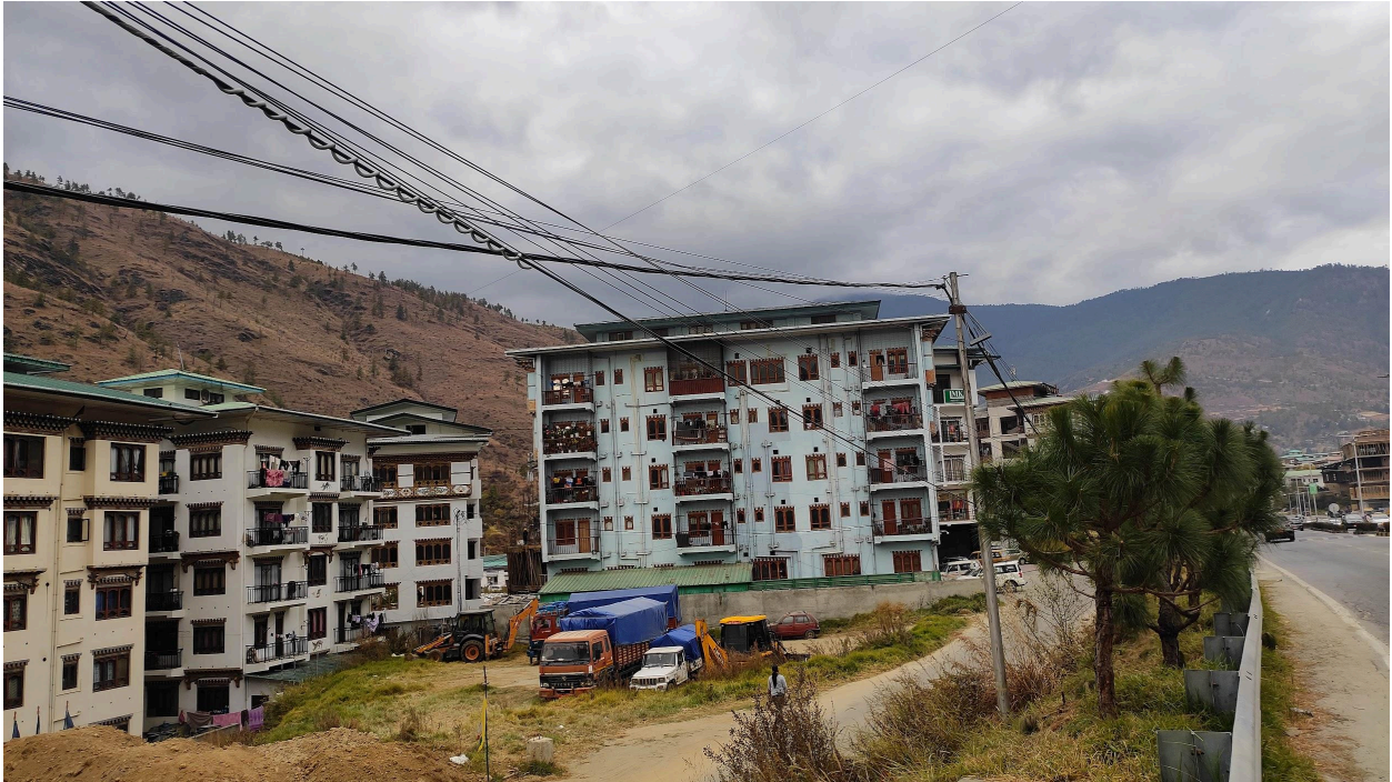
Figure 7 Improper cable layout along Babesa Express way, Before and After
