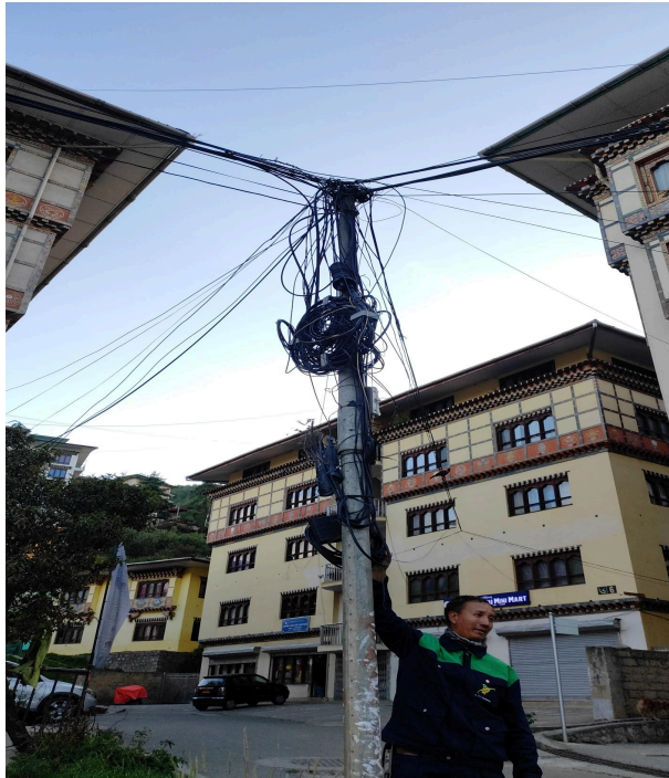
Figure 10: Improper crisscrossing of cables at Changbangdu, Before and After
