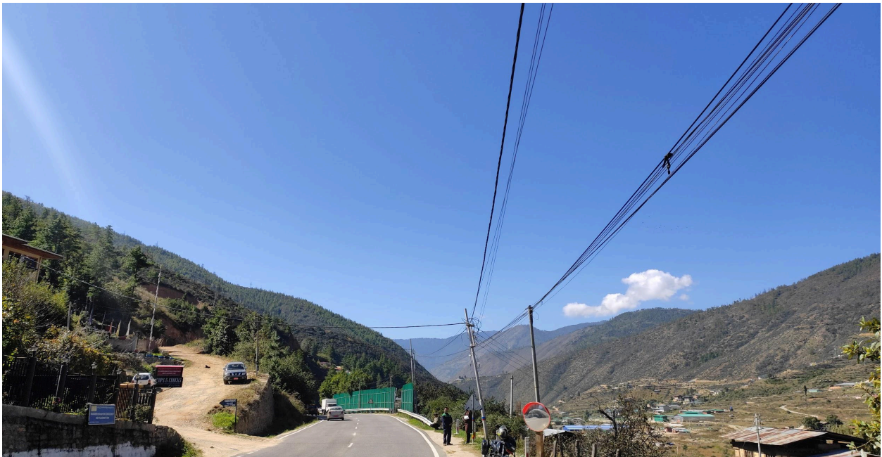
Figure 3: Improper Cable Layout; Before and After
