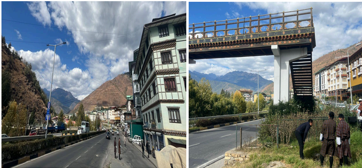
Figure 16: Common duct above Olakha workshop and towards Olakha Bridge
