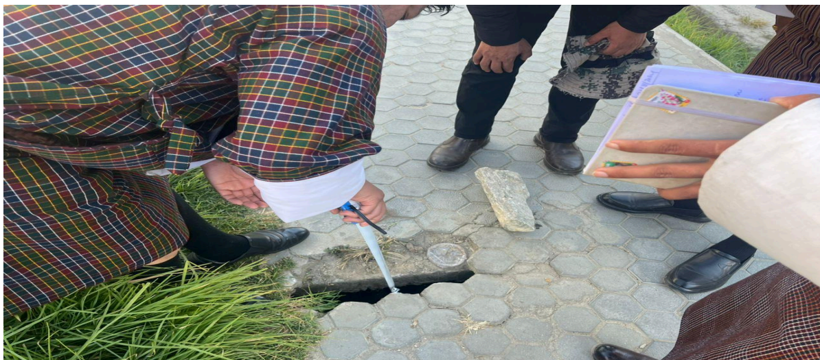
Figure 14: Common duct under the footpath along Babesa Express Highway
