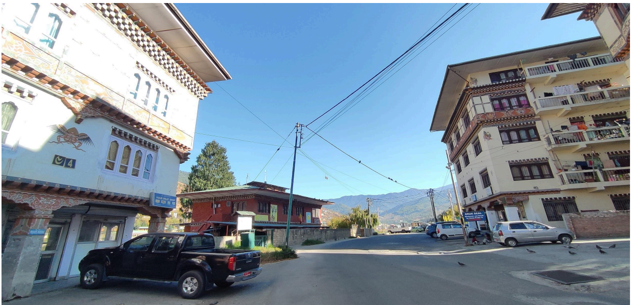
Figure 11: Improper cable road crossover at Changzamtok, Before and After
