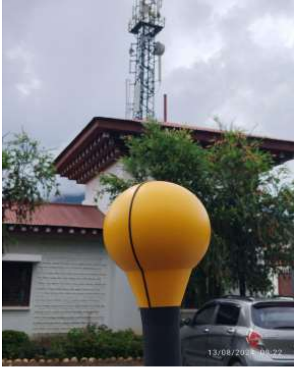
Figure 9: Wangdue Exchange (BTL)
