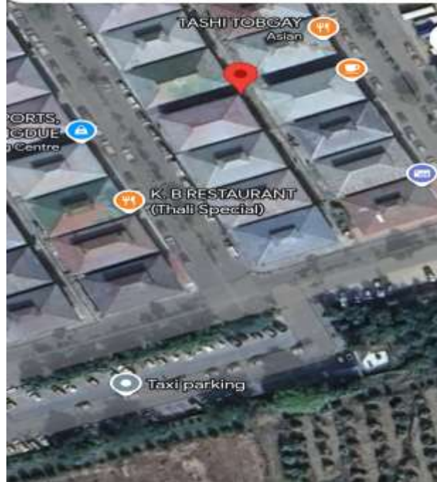
Figure 22: Bajo RoofTop, Wangdue (TIPL)
