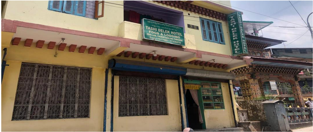
Figure 16: Proper layout of stray cable(RJ-6) near CableSat Office
